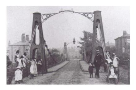
Here is a smaller suspension bridge. Can you see the deck? Can you see the cables and supports? The towers are right at the front of the picture. This little bridge did not cross to an island. It crossed a river. It made a way for people to get between two little towns. The towns were called Broughton and Pendleton. The rich man who owned the land had the bridge built. He wanted the little towns to have a grand bridge like Telford's. But this bridge was not so well built as Telford's bridge.
