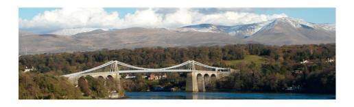
Have you ever seen a suspension bridge? "Suspension" means "hanging". A suspension bridge hangs from towers. The picture shows a suspension bridge. It crosses from the land to an island. The middle part is the hanging part. This part is called the deck of the bridge. This bridge was designed by Thomas Telford.
